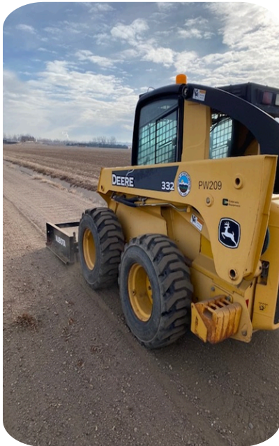
Wastewater- Streets crew using the box scraper to clean up the road
