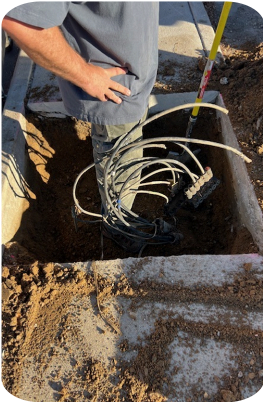
3RD Street- Sturgeon replaced the Quazite box with a new, more durable one.
