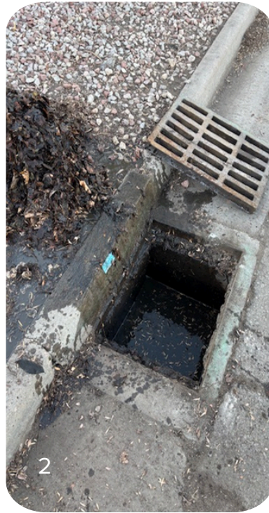
1 & 2) 1st Street- The Street crew cleaned out storm drain inlets 3) Bunyan Avenue- The Streets crew clearing excess snow from Bunyan Avenue
