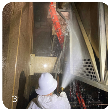
1) Caustic wall before repair 2) Caustic wall after repair 3 & 4) Sediment Basin Cleaning
