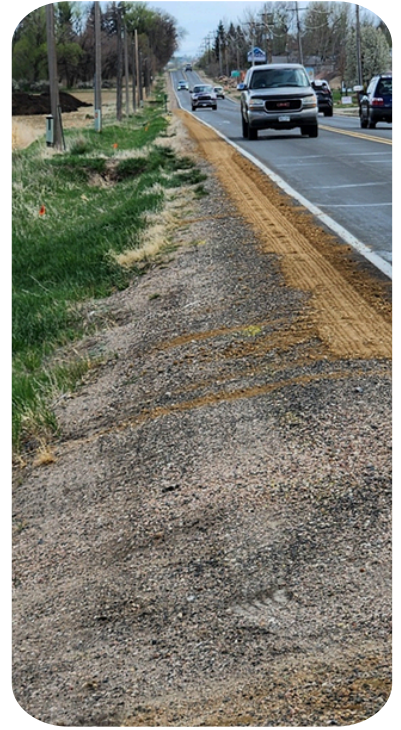
1st Street- The Streets crew is adding road base along sections of 1st Street to prevent water from pooling onto the roadside
