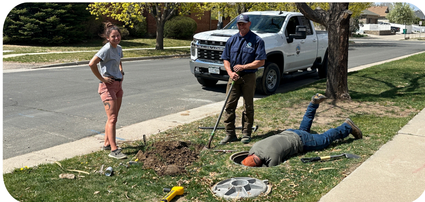
The Water and Parks teams work together to solve long buried pipe mysteries.
