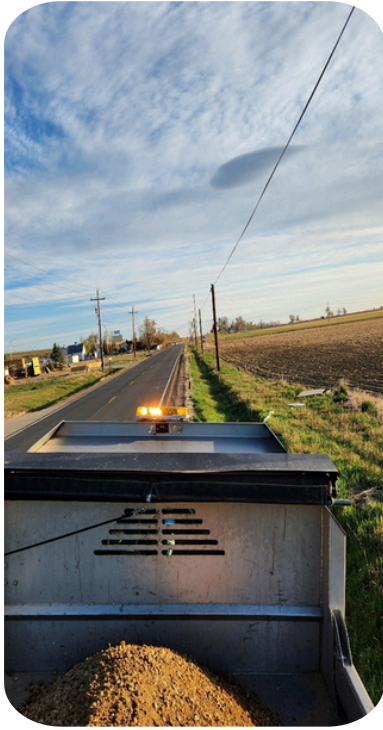
1st Street- The Streets crew is adding road base along sections of 1st Street to prevent water from pooling onto the roadside
