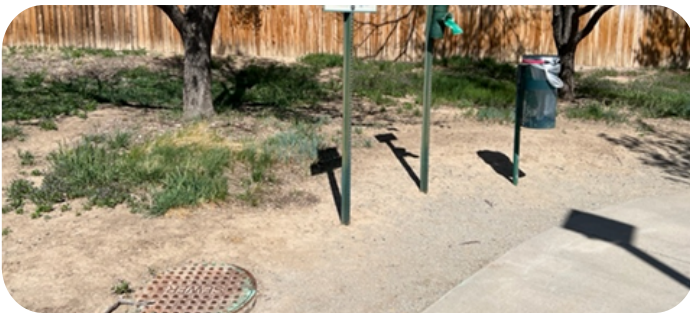
Working with the soil stabilizer used at the Bike Park, Open Space staff added some hard packed and stabilized crusher fines underneath the trash cans located along the Neilson Trail and along the walking trail just north of the Dog Park.
