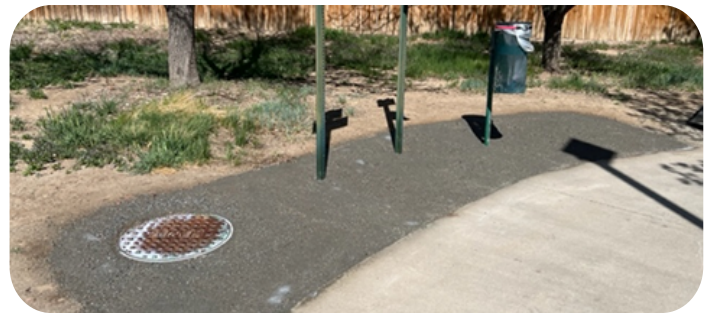
Working with the soil stabilizer used at the Bike Park, Open Space staff added some hard packed and stabilized crusher fines underneath the trash cans located along the Neilson Trail and along the walking trail just north of the Dog Park.
