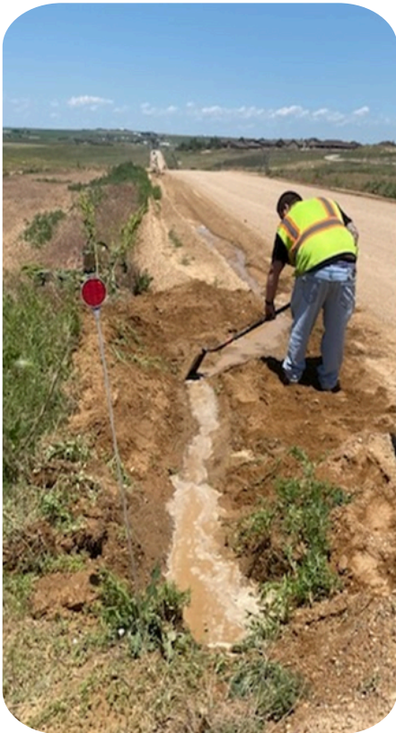
County Road 7- After the last major storm streets crew is cleaning out the culverts to make sure water can flow properly
