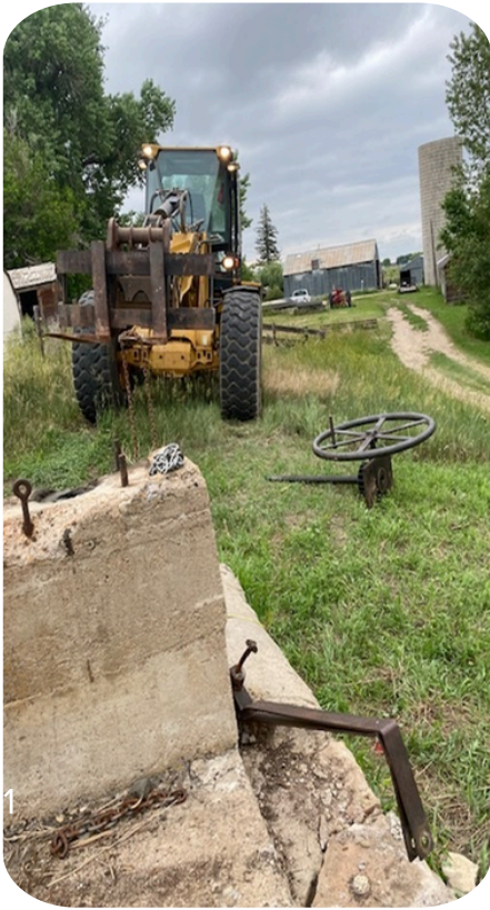
Loveland Reservoir- The Streets crew assisted the water department by removing the concrete section by the gate and installing a gantry so the gate could be opened by a hoist.
