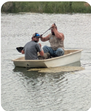
Open Space staff and Parks staff work together to install the aeration fountain in Pioneer Pond.
