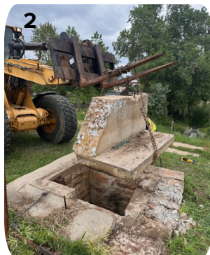
1) The gantry crane 2) Berthoud Streets Department removing the 3,000 lb cement block 3) The original hand crank wheel
