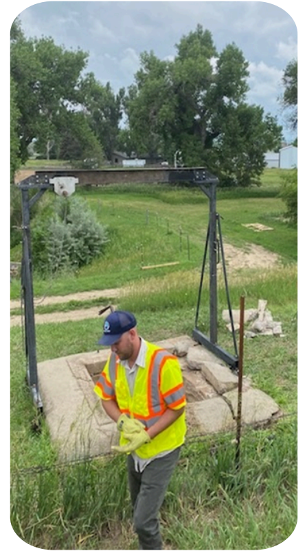
Loveland Reservoir- The Streets crew assisted the water department by removing the concrete section by the gate and installing a gantry so the gate could be opened by a hoist.
