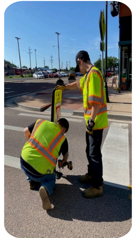
Mountain Avenue- Streets crew is installing pedestrian crossing signs in the center of the road to help motorists see pedestrians crossings
