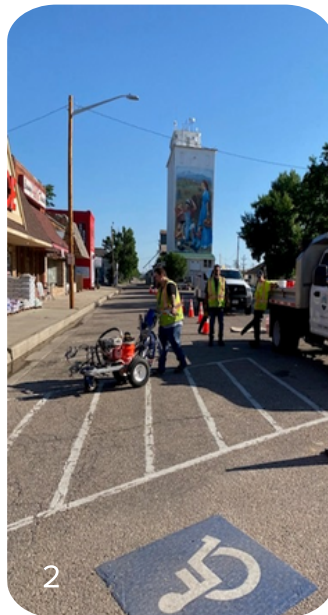
1 & 2) 3rd Street- Streets Department restriping parking stalls 3) Mountain Avenue- Streets Department setting out cones and barricades for the July 3 rd event 4) Bein Park -Streets crew helped the parks department dig around the irrigation lines so they could make repairs.
