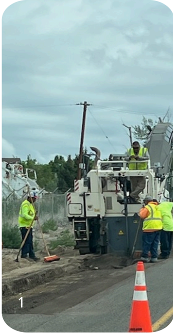
1 & 2) 1st Street- Goltz Asphalt Company is repairing sections of roadway that were failing. 3 & 4) 4 th Street- Goltz Asphalt Company is patching a section of roadway that was sinking
