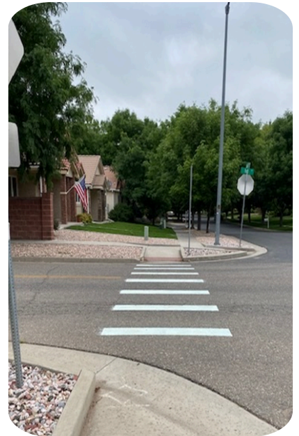
1st Street & Indiana- Streets crew replaced the crosswalk that was faded
