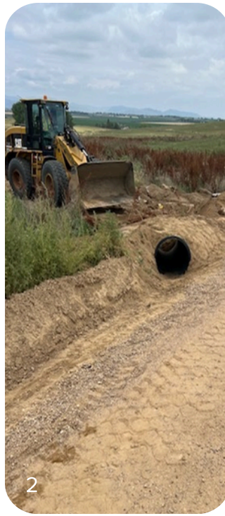
1 & 2) County Road 7- Streets crew cleaned out ditches and installed additional culvert pipes to divert water away from the roadway to help prevent erosion 3 & 4) Nielson drainage ditch- Streets crew jetting underneath box culverts to remove mud and debris
