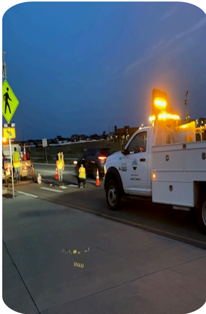
Berthoud Parkway & Grand Market- Streets crew came in early to repair crosswalk thermoplastics
