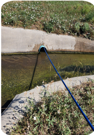
Robert's Lake- Streets crew jetting the storm drain outlet and cleaning the concrete channel
