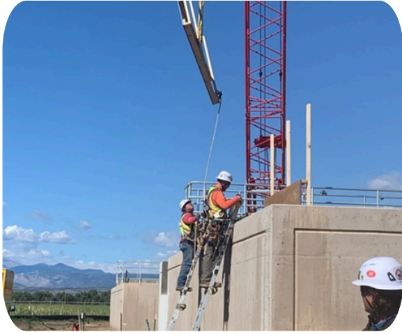
Staff setting forms for new ANA Basins
