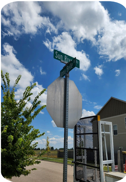
Vantage subdivision - Street crews installed new signage that blew off during a strong windstorm.
