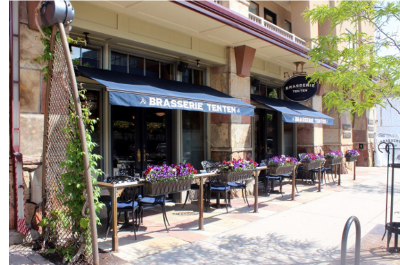
Private encroachment dining & furniture
