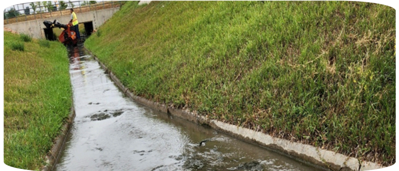
Nielsen Drainage - Street crews cleaned all the moss off the concrete in the drainage channel.
