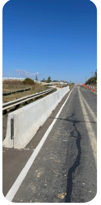
Jersey barriers were added on Berthoud Parkway to protect pedestrians on the trail.
