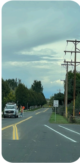
Meadow Lark Drive - existing lane stripes were removed and reconfigured to make room for bike lanes.
