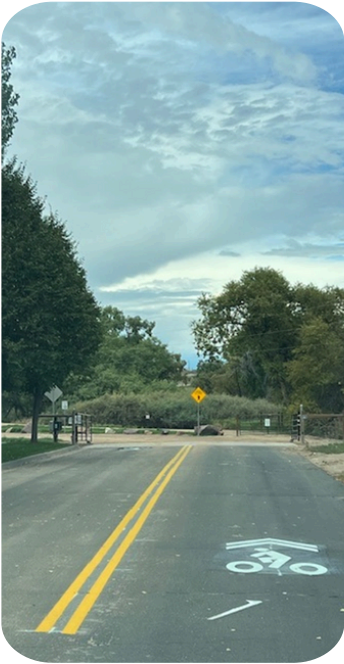
Meadow Lark Drive - existing lane stripes were removed and reconfigured to make room for bike lanes.
