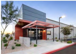
PRIMARY BUILDING ENTRANCE
