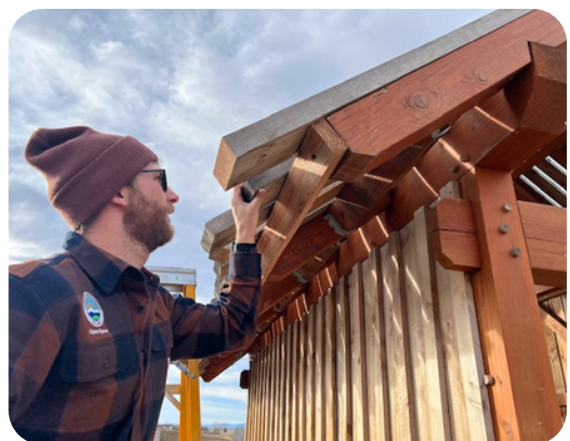
Open Space staff repaired a broken board on the roof of the “Shred Shed” at Berthoud Bike Park and reinforced the landing area with extra supports to hopefully eliminate future breaks.
