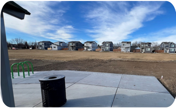
Earthworks were completed at Pioneer Park, making it ready for the new pickleball court.
