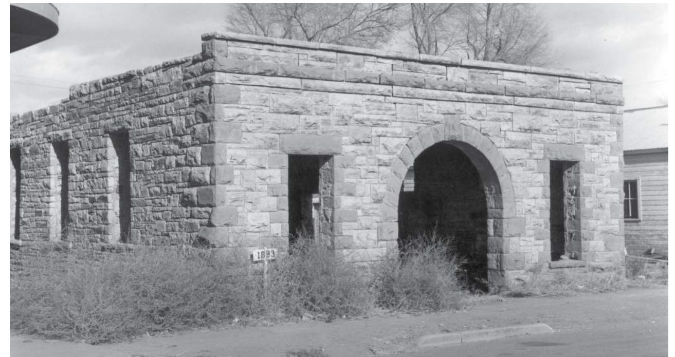
Bimson's Blacksmith Shop prior to its purchase and rehabilitation by the Berthoud Historical Society. Today the organization runs the little Thompson Valley Pioneer Museum out of the building. The blacksmith shop is listed on the National Register of Historic Places. (Source: Library of Congress)
