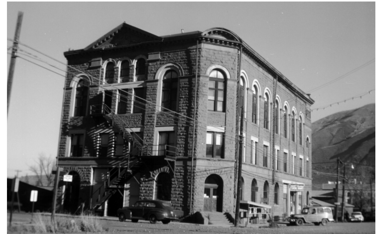
The Wheeler Opera House, pictured here in 1957, received a preservation award from Aspen's City Council in 2023 for a significant exterior renovation which included replacement of its sandstone exterior sourced from a quarry in Wyoming.
