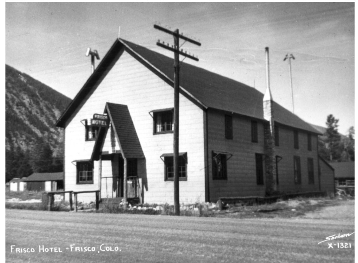
Historic resource surveys identify and evaluate historic properties in a community, such as the historic Frisco Hotel, pictured here in the early 1900s.
