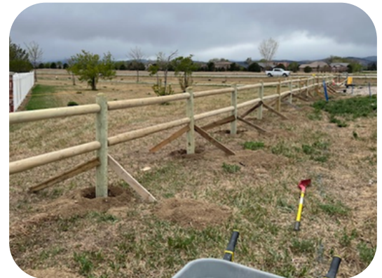
Crews reinforced the fence at Berthoud Bike Park.
