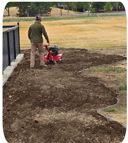
Landscaping work has begun at the Pioneer Park Pickleball court.
