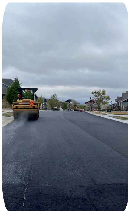
Crews have been working to repair Tipton Street.
