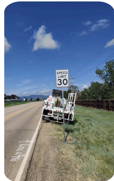
County Road 14- Street crew installed a new 30mph sign after it was struck by a vehicle
