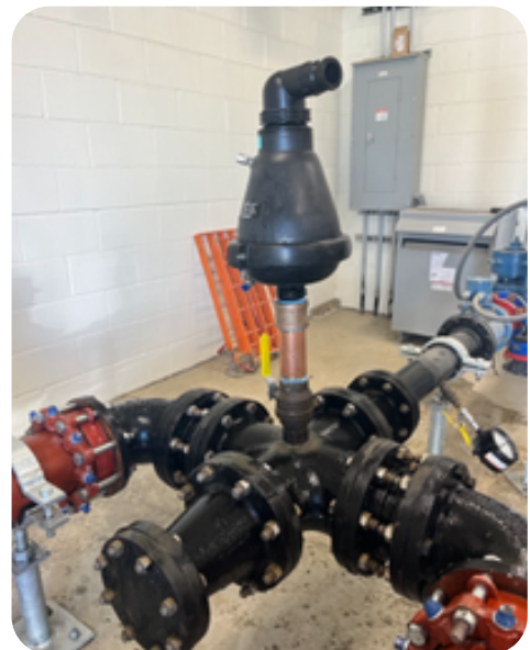
AirVac Replacement – Heron Lakes Lift Station
