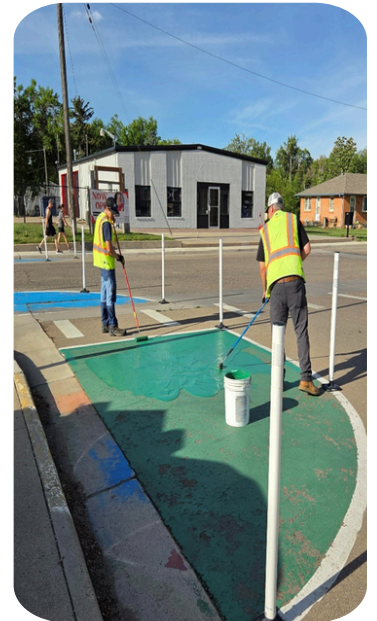
3rd St. & Welch Ave.- Streets crew refreshed the tactical urbanism with new paint
