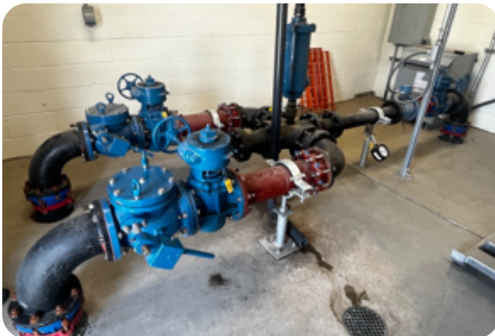
AirVac Replacement – Heron Lakes Lift Station
