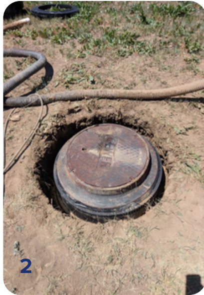
1) Manhole Raise – Valleyview 2) Manhole Raise – Valleyview 3) Manhole Raise – Valleyview
