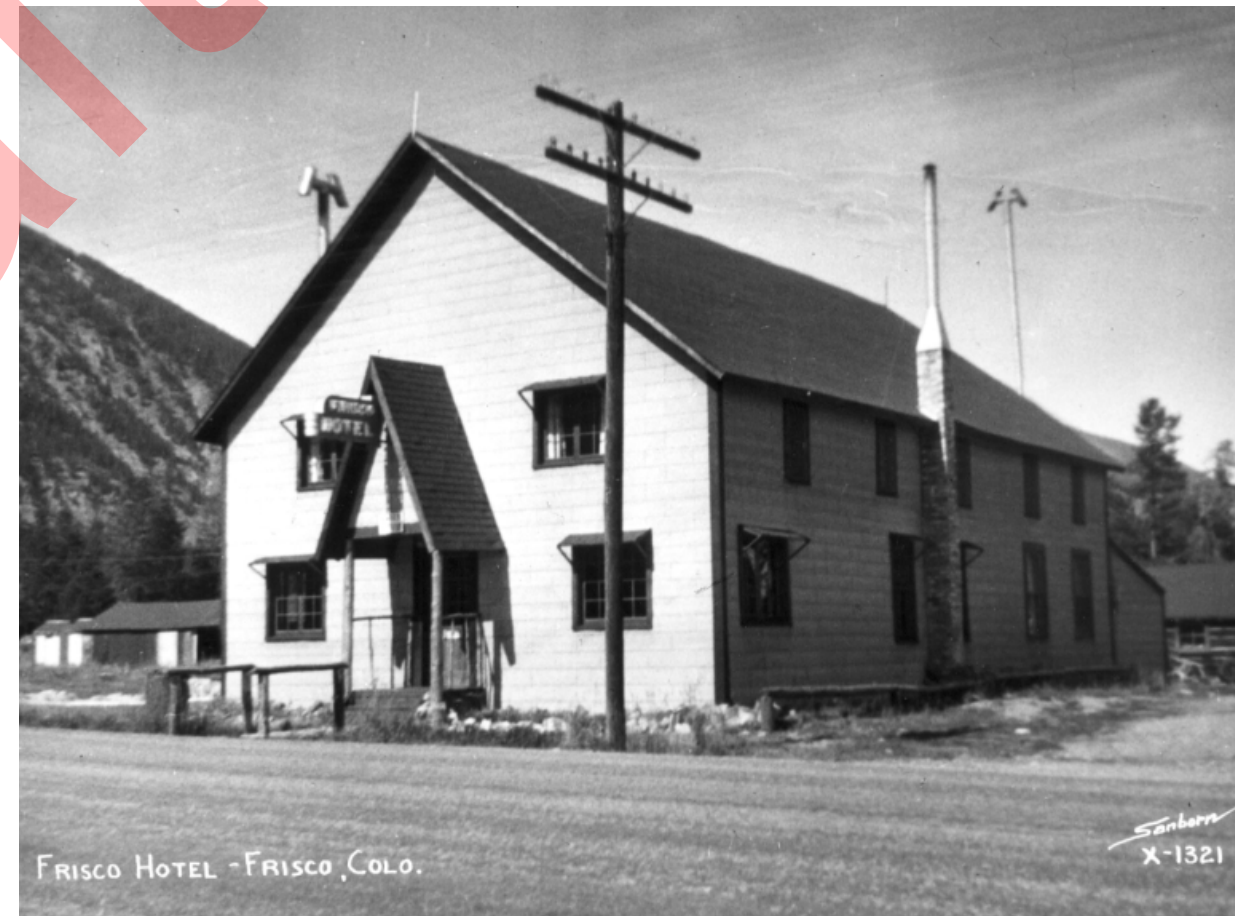
Historic resource surveys identify and evaluate historic properties in a community, such as the historic Frisco Hotel, pictured here in the early 1900s.
