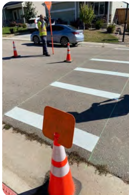
Prairiestar Dr. Crosswalk installed
