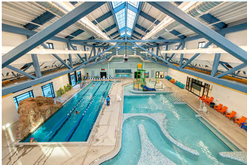
The pool at Berthoud's award-winning Recreation Center
