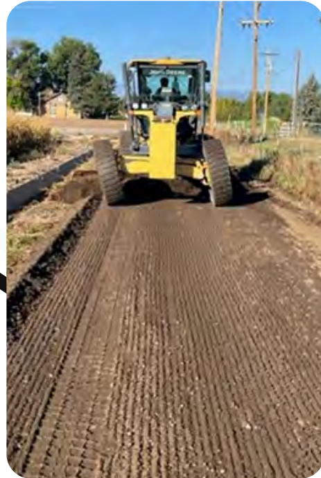
Grading the Wastewater Plant entrance road
