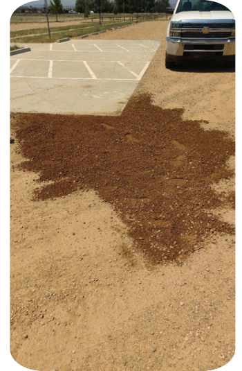
Berthoud Recreation Center- Streets crew placed road base next to the parking stalls and sidewalk to help reduce tripping hazards
