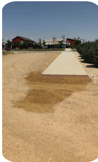
Berthoud Recreation Center- Streets crew placed road base next to the parking stalls and sidewalk to help reduce tripping hazards
