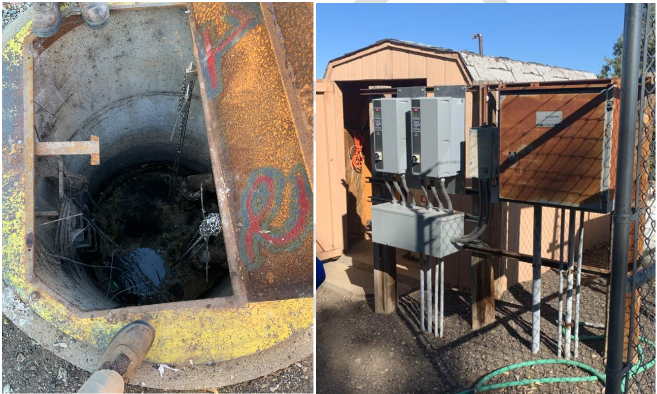
Figure 5-25: WWC-5: Bomar Lift Station Upgrades – Existing Conditions
