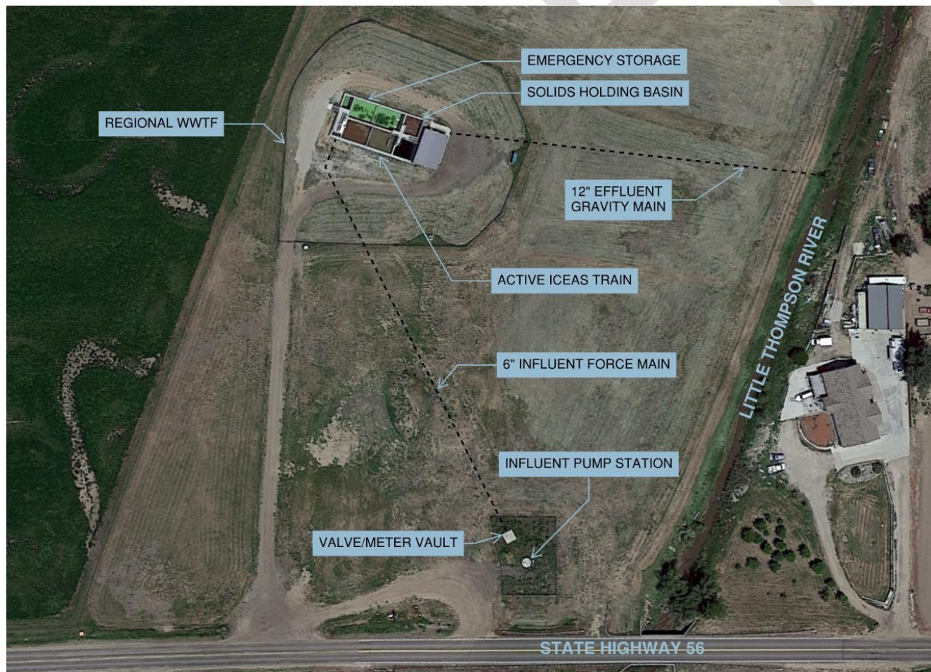
Figure 5-9: Regional WWTF and Influent Lift Station
