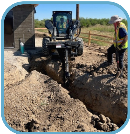
Bike park- Streets crew trenched ditches for the installation of electrical lines
