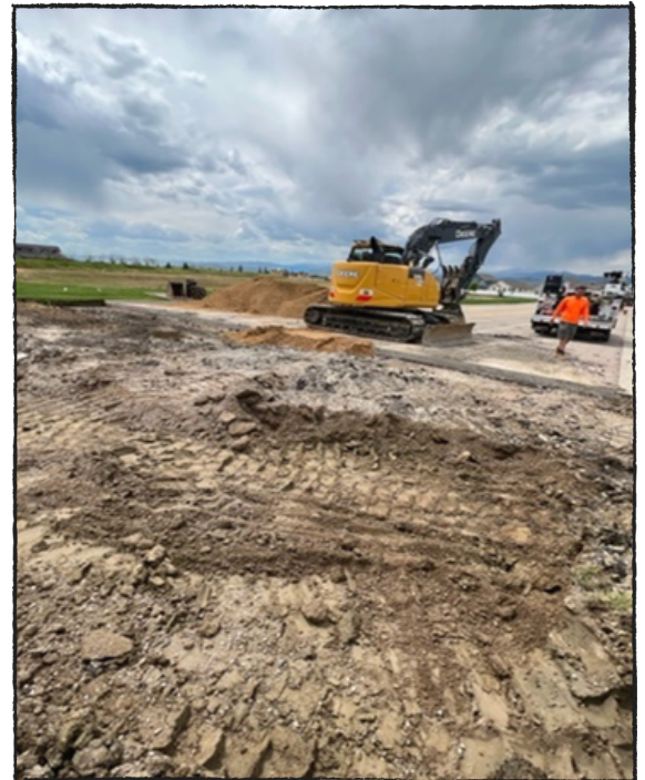
County Road 10E- Gopher excavated the site of the sinkhole and determined that it was caused by water infiltration and poor subgrade compaction in the past.
