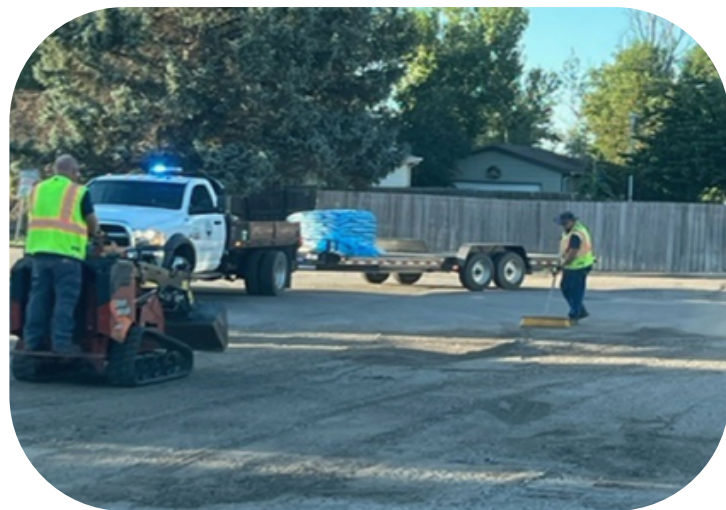
2nd Street- Streets crew cleaning up loose millings and filling potholes with cold patch
