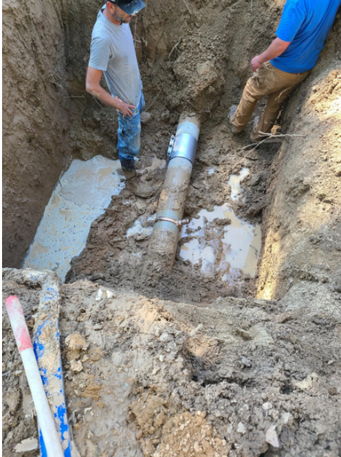
Helping to repair a service line break in Town Park.
