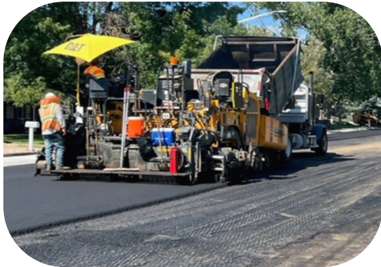
Oldtown- The road on 6th Street is currently undergoing milling and receiving an asphalt overlay
