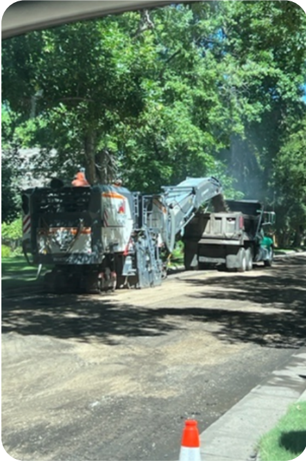
Oldtown- The road on 6th Street is currently undergoing milling and receiving an asphalt overlay
