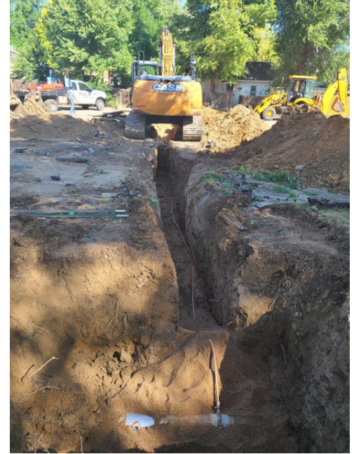
Helping to repair a service line break in Town Park.
