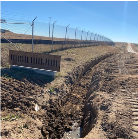
County Road 7- The streets crew dug a ditch to help with drainage coming from Ball Aerospace Drive.
