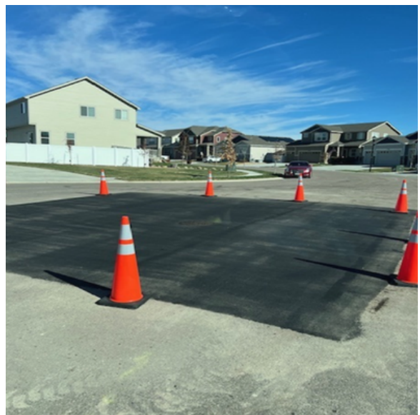
Hammond Farms- There was sinking around the manhole on Cadman Street, so excavation work was performed as well as an asphalt patch.
