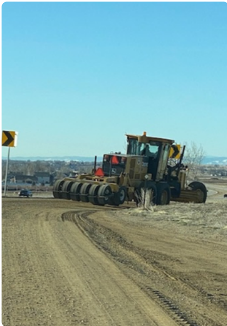
Streets crew grading county road 10E
