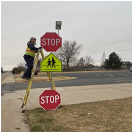
Flashing stop signs installed at Ivy Stockwell
