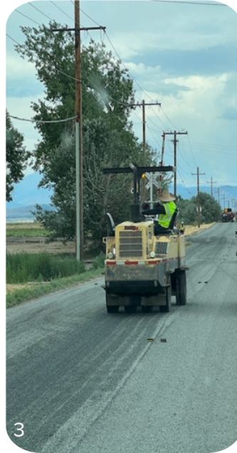
1. Dust suppressant being applied to CR10E 2. Grading wastewater road 3. County Road 10E and Water Ave are crack-sealed, and chip-sealed 4. Filling in the potholes and smoothing out the alleys in Oldtown
