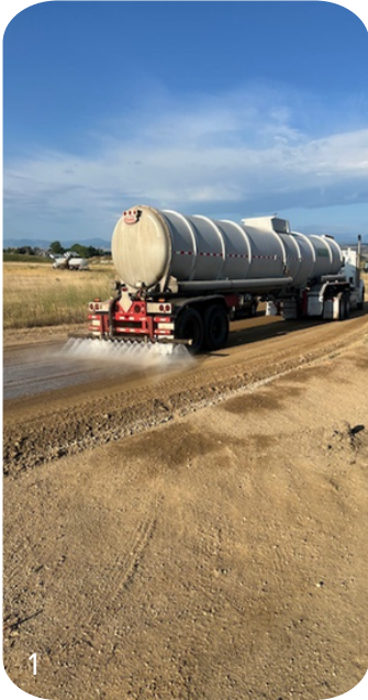
1. Dust suppressant being applied to CR10E 2. Grading wastewater road 3. County Road 10E and Water Ave are crack-sealed, and chip-sealed 4. Filling in the potholes and smoothing out the alleys in Oldtown
