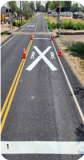
1 & 2. CR10E- After striping was completed, railroad crossing and thermoplastics turn arrows were installed 3. Streets Crew teamed up both sweepers to do a thorough cleaning of downtown 4. Streets crew mowed the field on the Richardson property
