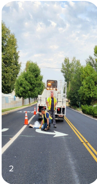
1 & 2. CR10E- After striping was completed, railroad crossing and thermoplastics turn arrows were installed 3. Streets Crew teamed up both sweepers to do a thorough cleaning of downtown 4. Streets crew mowed the field on the Richardson property
