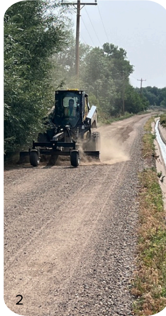
1. Dust suppressant being applied to CR10E 2. Grading wastewater road 3. County Road 10E and Water Ave are crack-sealed, and chip-sealed 4. Filling in the potholes and smoothing out the alleys in Oldtown
