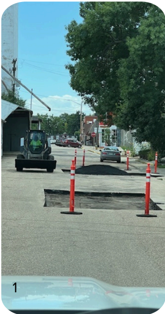
1 & 2 - Patching sunken areas on 3rd St. There were a total of 17 patches 3&4 - Streets crew installed new type 3 barricades at the dead end of SE 3rd Street and East Michigan Avenue.
