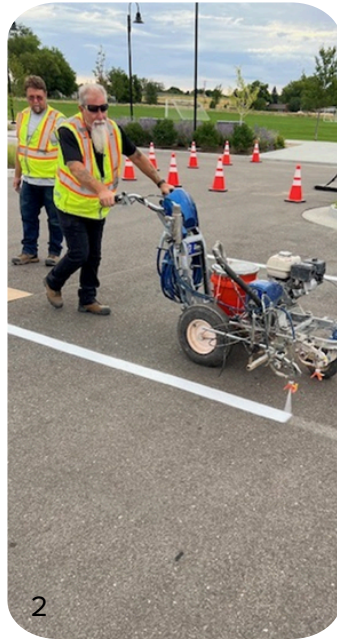
1 - Restriping curbs at Turner Middle School 2 & 3 - Restriping parking stalls at the Recreation Center 4 - Restriping parking stalls on 3rd St.
