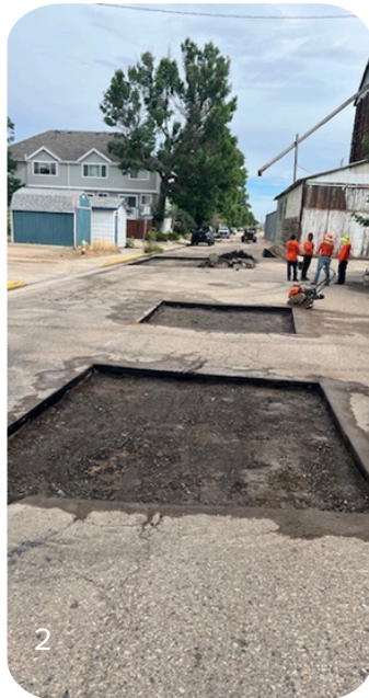
1 & 2 - Patching sunken areas on 3rd St. There were a total of 17 patches 3&4 - Streets crew installed new type 3 barricades at the dead end of SE 3rd Street and East Michigan Avenue.
