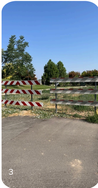
1 & 2 - Patching sunken areas on 3rd St. There were a total of 17 patches 3&4 - Streets crew installed new type 3 barricades at the dead end of SE 3rd Street and East Michigan Avenue.
