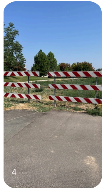
1 & 2 - Patching sunken areas on 3rd St. There were a total of 17 patches 3&4 - Streets crew installed new type 3 barricades at the dead end of SE 3rd Street and East Michigan Avenue.
