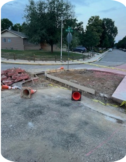
3rd and Indiana- Lucero concrete removed and replaced the concrete median as well as the curb and gutter
