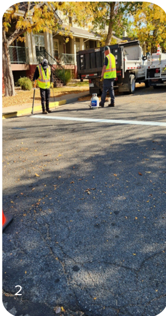
1) The Streets Department repainted the tactical urbanism on 3rd street 2) installing new stop bars along Welch Ave. 3 & 4) installed a new pedestrian crossing on Greenwood Drive to accommodate the walking trail, following a request from a resident.
