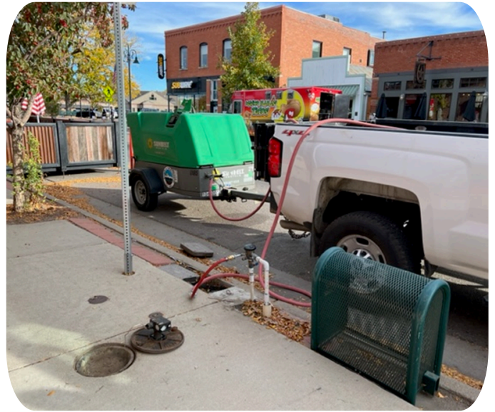
Annual pots were removed on Main Street and the irrigation systems were winterized in October.
