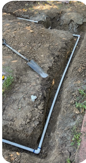
The Community Garden on the west side of Pioneer Park has been undergoing upgrades to enhance the space. One such upgrade has been the irrigation. The system used to run off only two valves, but an additional valve was added to accommodate more garden beds, and new irrigation piping was laid to get water to every bed, tree and bush in the garden.
