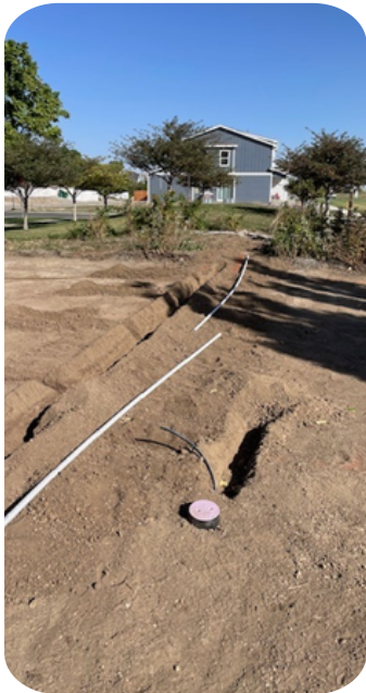
The Community Garden on the west side of Pioneer Park has been undergoing upgrades to enhance the space. One such upgrade has been the irrigation. The system used to run off only two valves, but an additional valve was added to accommodate more garden beds, and new irrigation piping was laid to get water to every bed, tree and bush in the garden.
