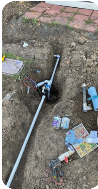
The Community Garden on the west side of Pioneer Park has been undergoing upgrades to enhance the space. One such upgrade has been the irrigation. The system used to run off only two valves, but an additional valve was added to accommodate more garden beds, and new irrigation piping was laid to get water to every bed, tree and bush in the garden.
